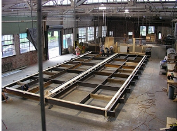
Figure B – Steel Frame Platform
